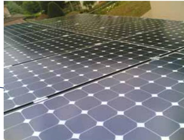
Black, back contact monocrystalline cells - **aesthetically more pleasing** for architectural installations. High efficiency for maximum energy yield per square metre.
